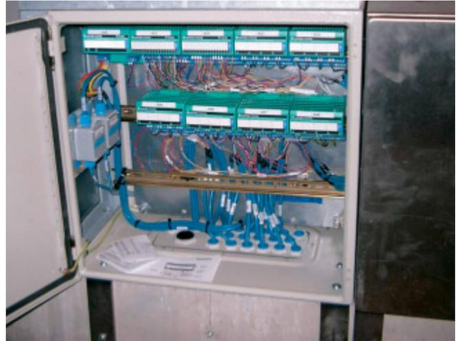
Figure 8: IS-RPI in the switch cabinet.
